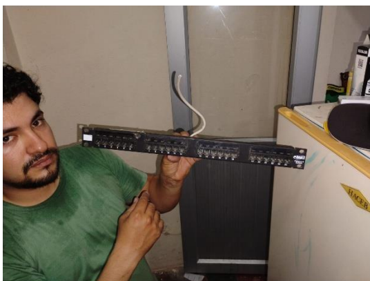
Figura 12. Poe (Power over Ethernet)
